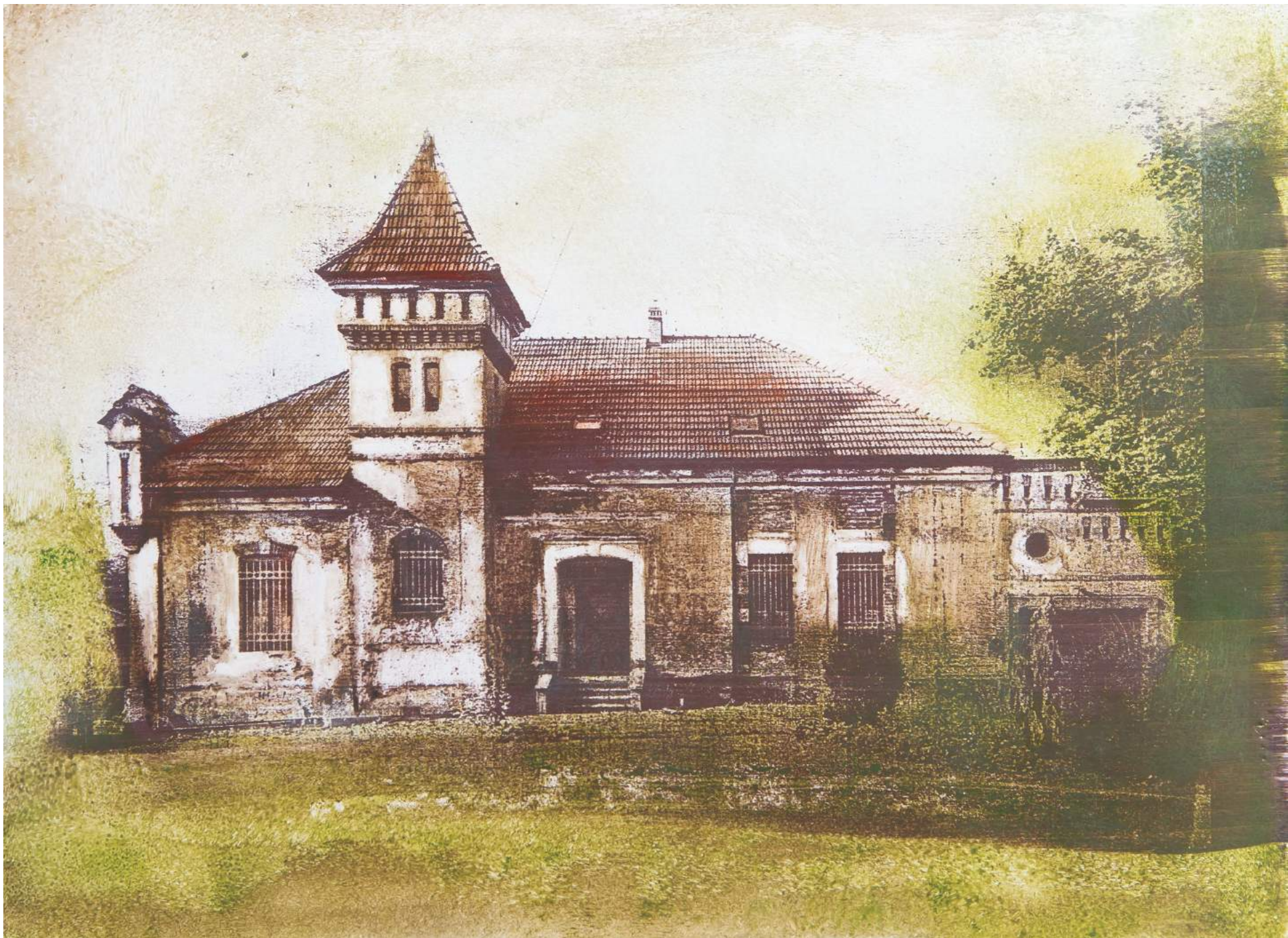
dwór w Boleniu / manor house in Boleń
