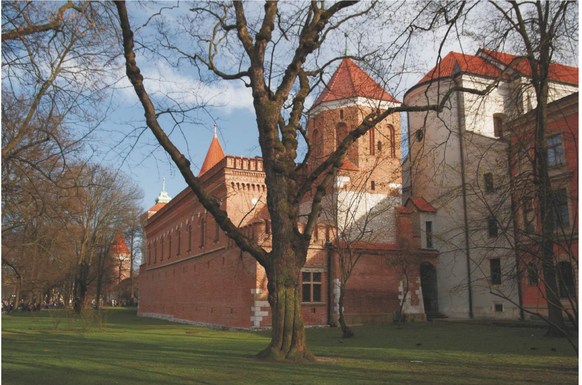
baszty i mury obronne starego miasta / towers and defence walls of the old town
